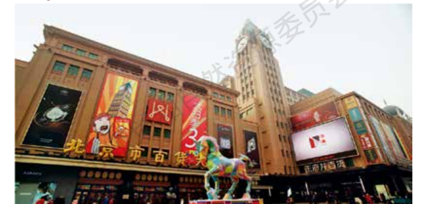
改造前：广告大面积遮挡建筑立面（全景网提供） Before renovation: disorganized advertising on building facade
