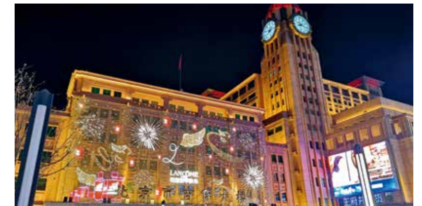
改造后：拆除广告，亮出建筑立面（辛萍摄） After renovation: advertisements dismantled and facade of the building revealed
