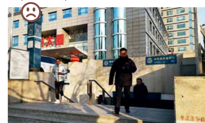
西钓鱼台地铁站 A 口：敞口式站口，无遮蔽设施 (辛萍摄) Exit A of Xidiaooyutai Station: An open station with no shelter
