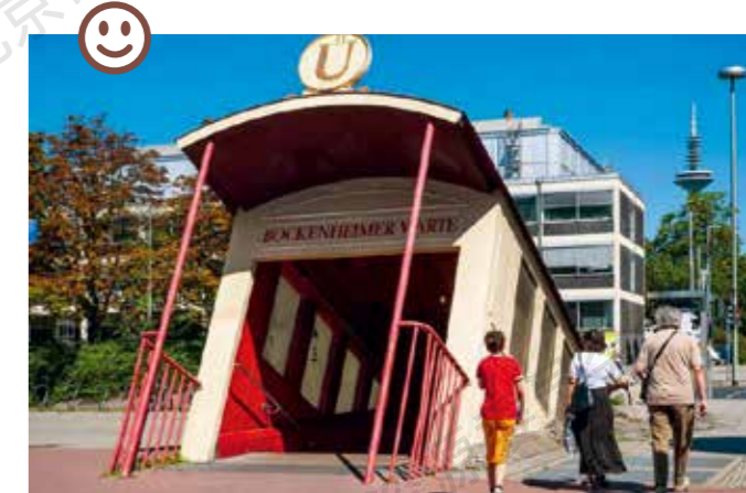
德国某地铁站：敞口式地铁站口上方设置雨棚 (全景网提供) A subway station in Germany: A rain canopy above the open station
