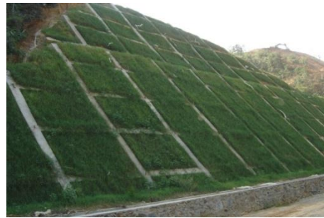
7-2 锚杆框架防护
