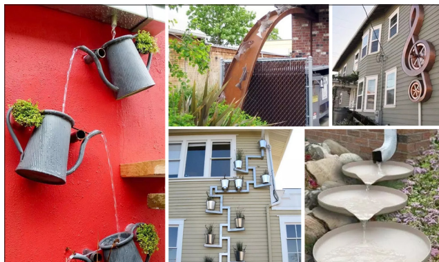
图7 景观化屋顶雨水管断接建设效果 Fig.7 Landscape-oriented disconnected rainwater pipes
