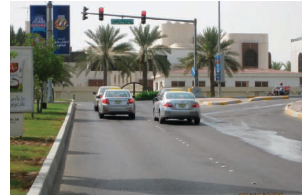
The Manual will emphasize the use of signalized junctions and pedestrian crossings in order to maximize safety.
