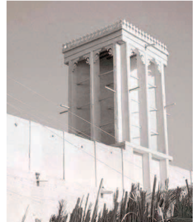
Historical photograph showing wind capture through the use of a wind tower, integrated in a sikka.
