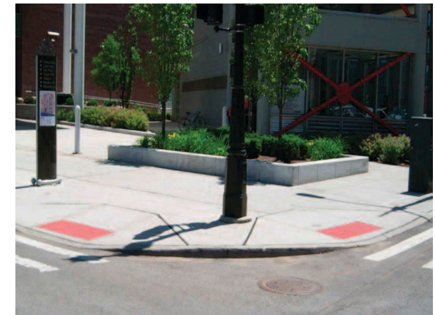
Curb ramps with detectable warning strips.
