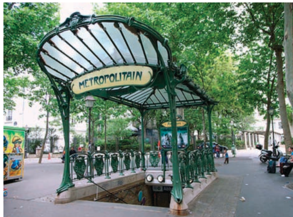
High quality Metro station entrance, Paris, France.
