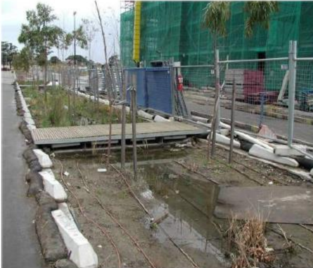
Figure 5-1 Example of Building Phase Destruction of a Bioretention Swale
