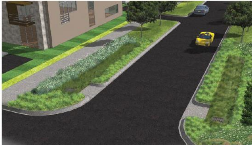
Figure 18 — Bioretention is clustered at the entry to the local access street. The figure also illustrates the preferred allotment orientation adjacent to entry points to local access streets on flat sites. A typical application of bioretention to the road verge for stormwater treatment is also shown.
