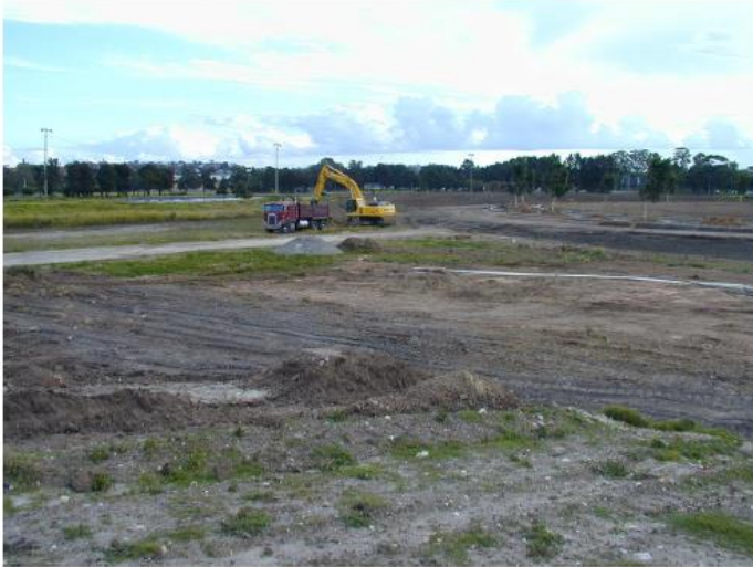
Wetlands site – construction beginning 2001
