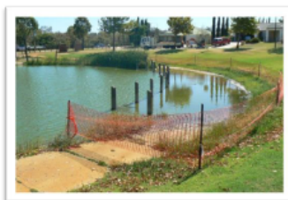
Parkfield Lake was previously subject to flooding and dangerous algal blooms
