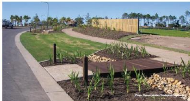
Example of WSUD street layout 2: Bioretention swale located on the high side of street (note the minimal number of driveway crossovers)
