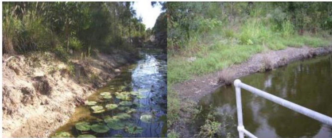
Figure 5-2 Examples of Erosion within Constructed Wetlands
