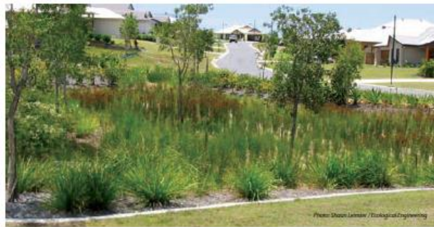
Example of WSUD street layout 1: Bioretention system in local park on the low side of street
