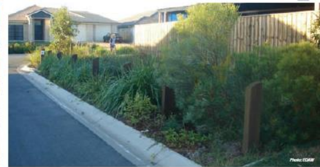
Example of WSUD street layout 3: Bioretention 'pod' located within street verge
