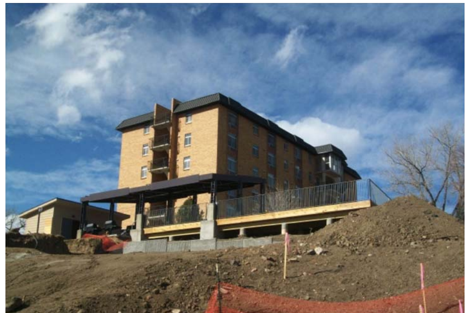
Deck trellis under construction at the Mulroy Apartments near the Knox station. This complex is managed by the Denver Housing Authority.
