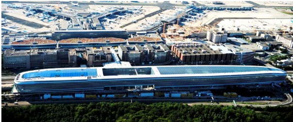
The squire, a groundscraper located in Francfort Airport City (Hub of Star Alliance), is one of the largest office building in Germany and use by Fraport to attract international companies such as European activities of KPMG.
