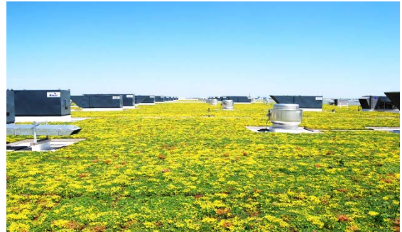
Green roof at Chicago airport © tcooper1960
