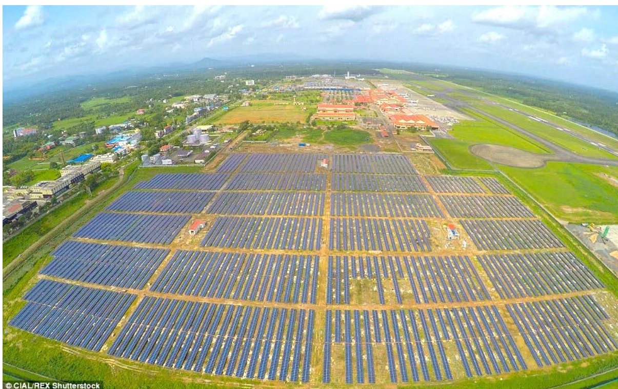
© CIAL/REX Shutterstock Cochin International Airport solar power plant, India
