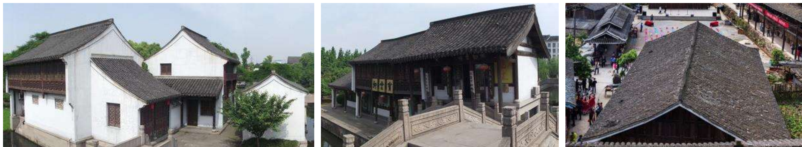
“人”字形坡屋顶
